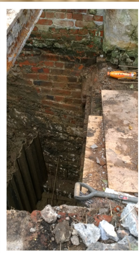
Southern side of headrace showing exposed brick and chalk courses
