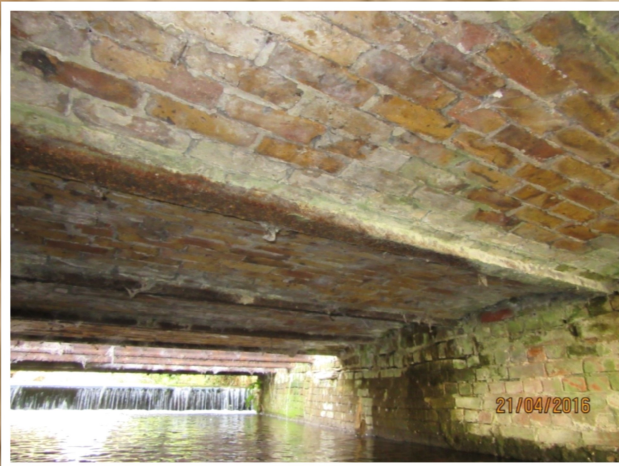
Jack arch above head race before removal
