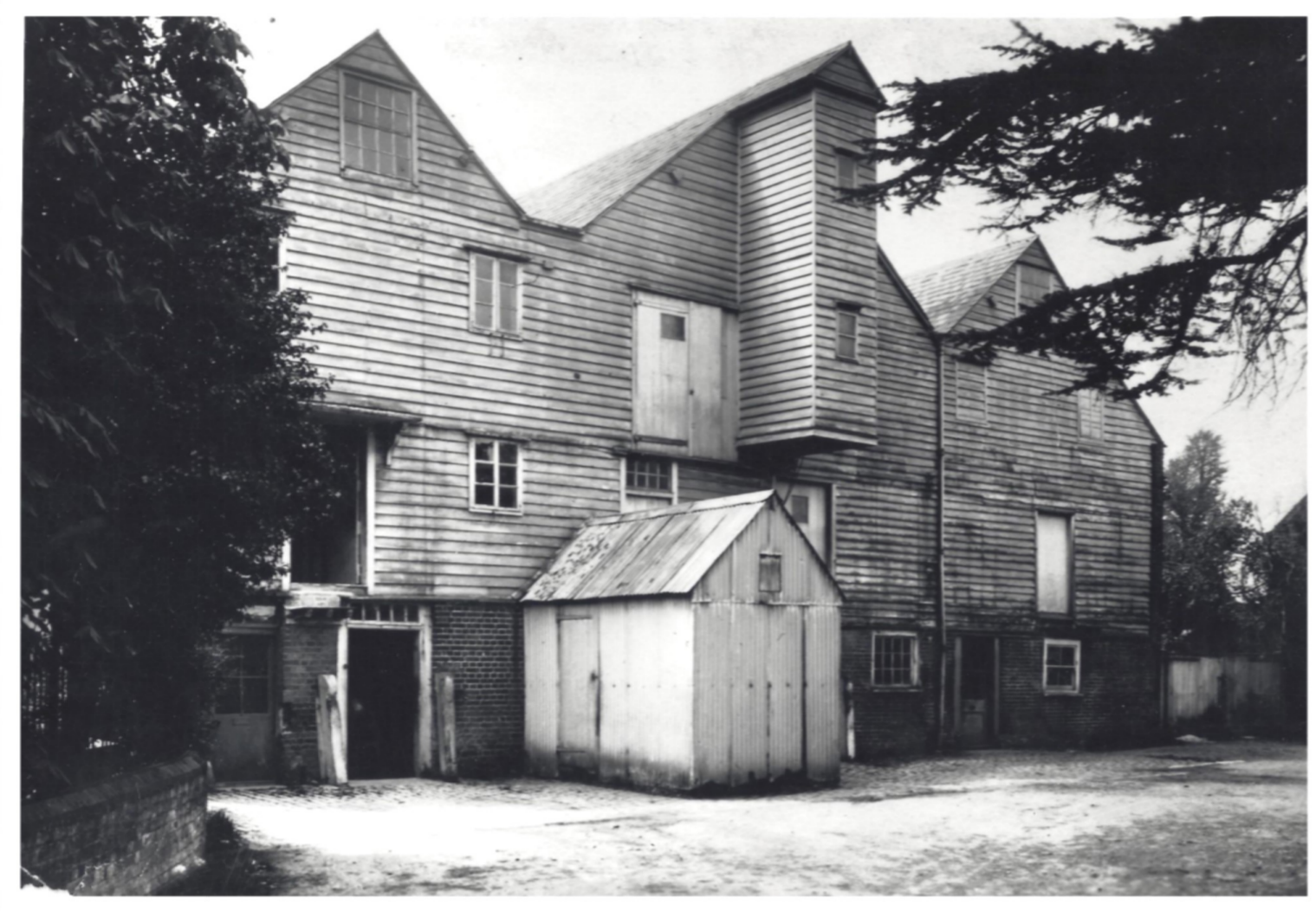
The Upper Mill, northern elevation with stables on the right, 1929
