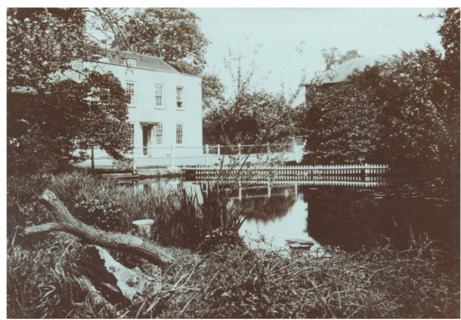
The miller's house at Lower Mill, 1920s
