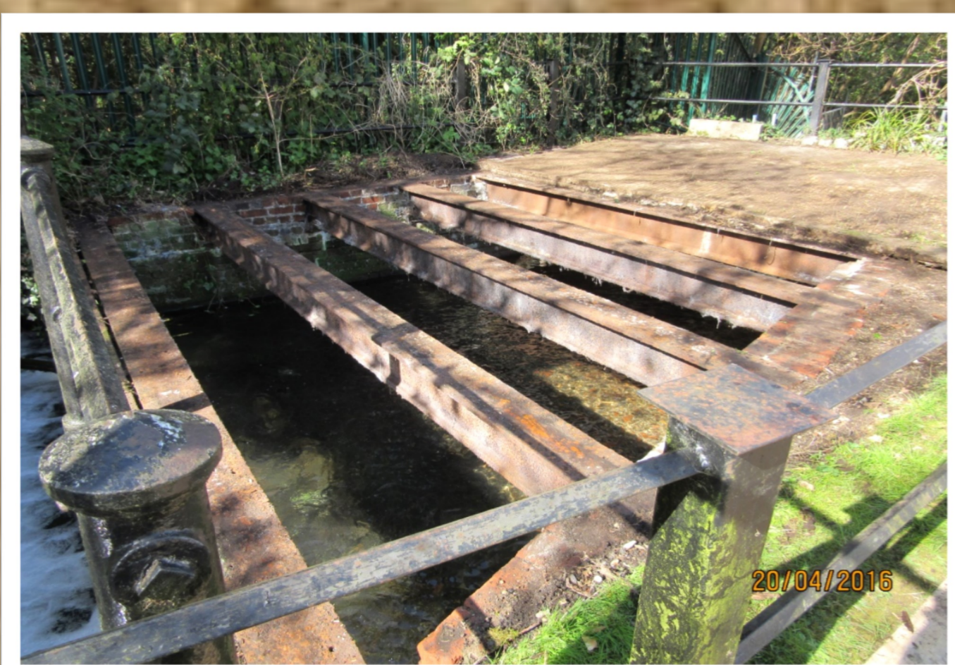
View of girders across the headrace
