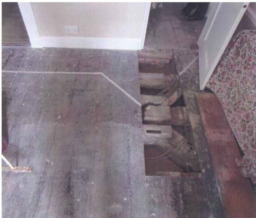
Floor construction under ground floor front room showing original octagonal form
