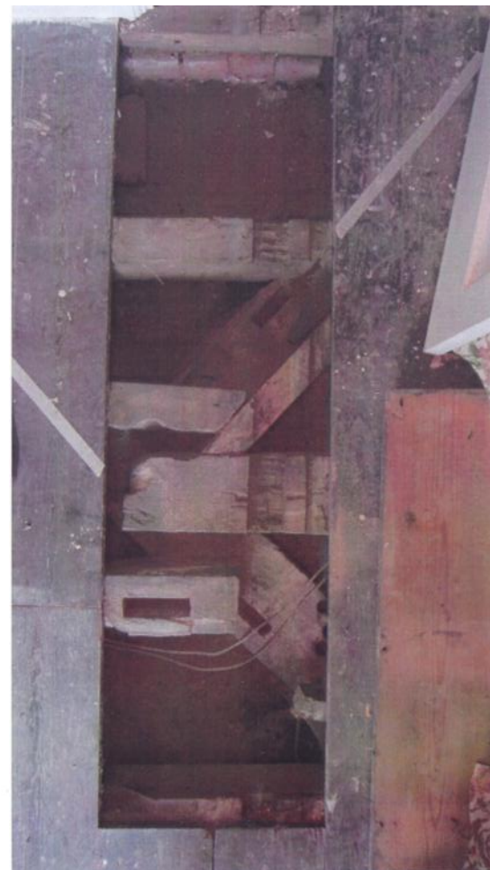
Floor construction under ground floor front room showing original octagonal form
