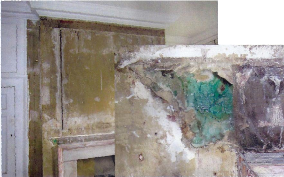
Front ground floor with fragment of c18 wallpaper behind fireplace surround
