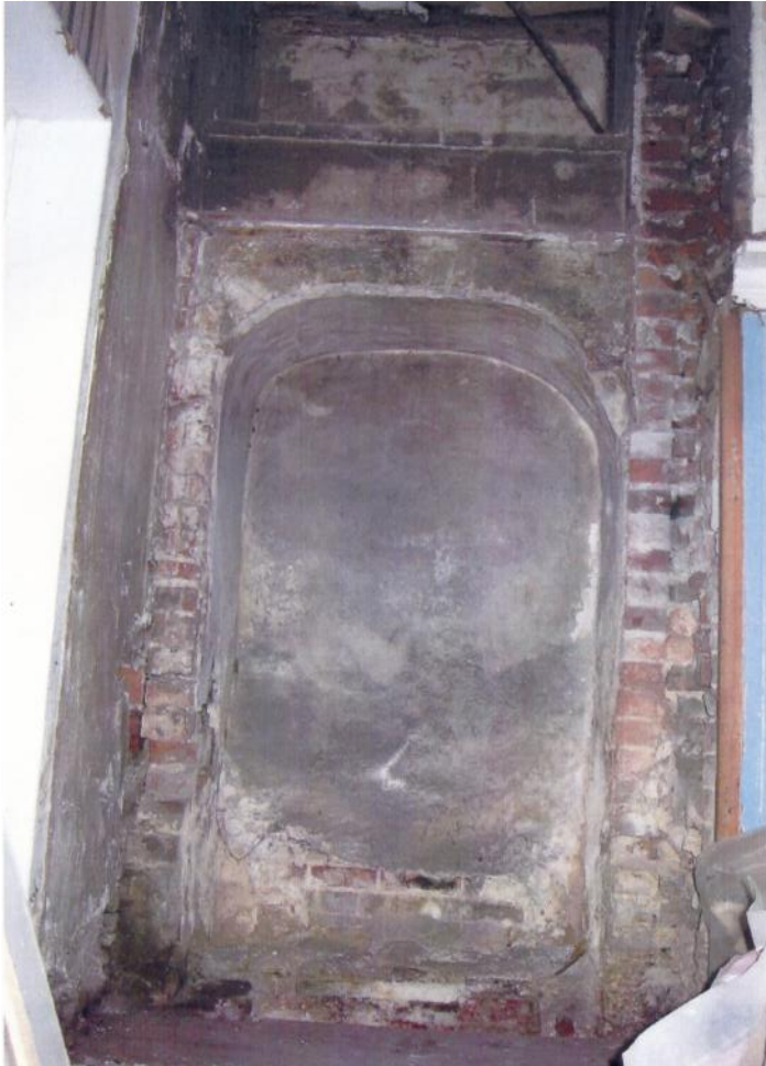
Voids found beside fireplace in kitchen which would have housed a lead water tank.
