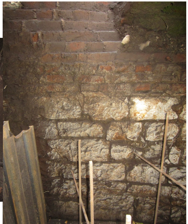
South wall: Original chalk block and two phases of brickwork
