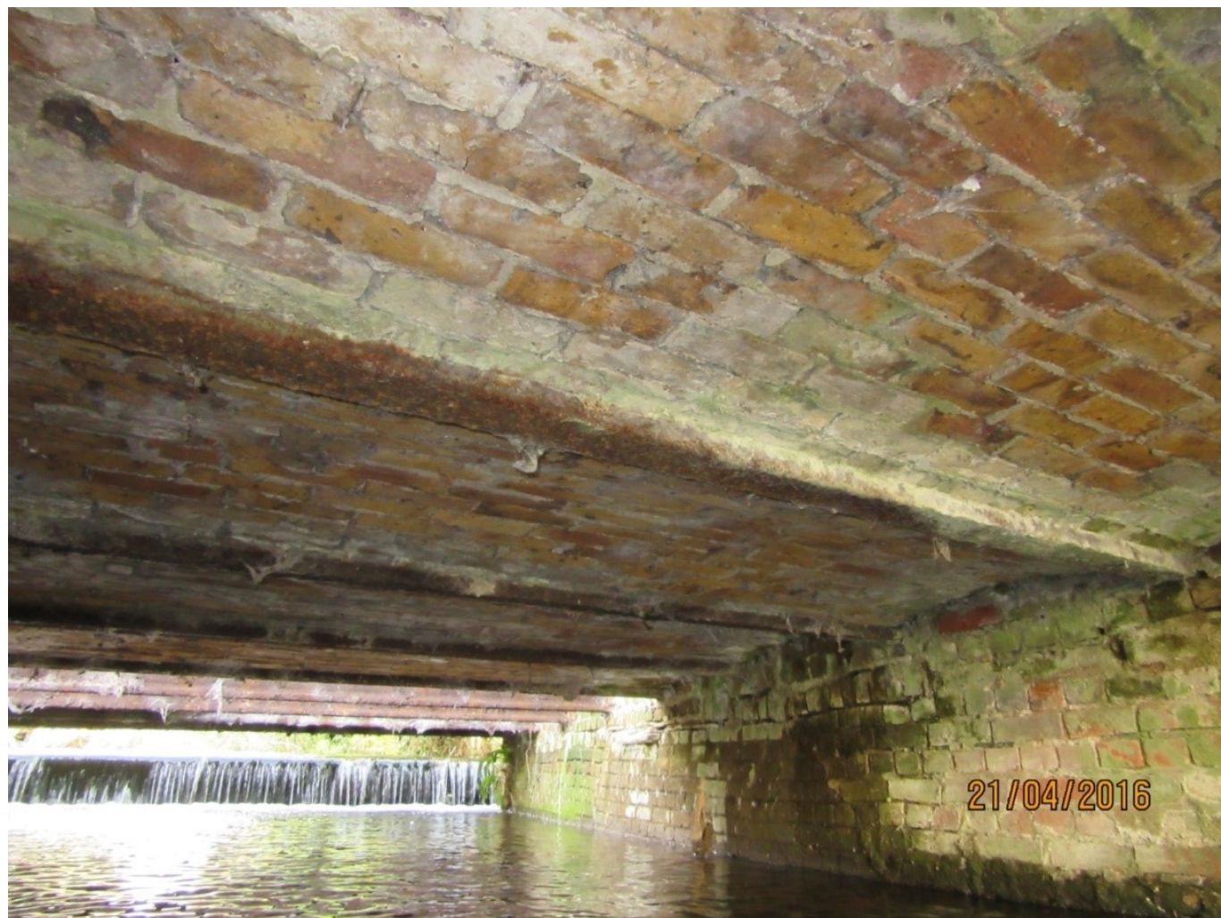
Jack arches above head race before removal
