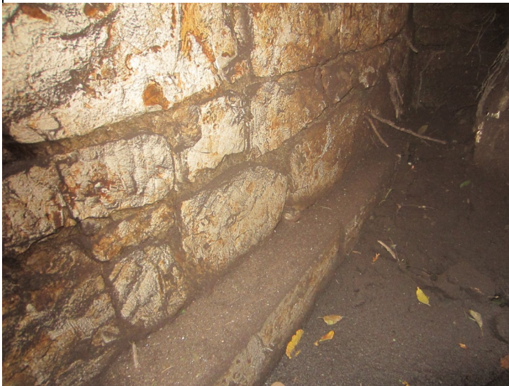
South wall: Chalk block with offset plinth at base
