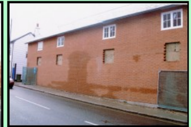
The replacement wall under construction
