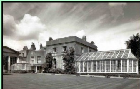
Below- Pitt Place, Church Street, Epsom prior to demolition
