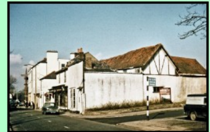
Nuttall's shop at 5-5a Cheam Road, Ewell- a 16th century jettied building demolished in 1968
